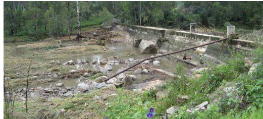
Below the wall of Dam 3a
